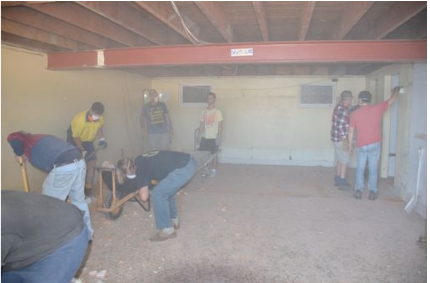
Demolition in progress. Many hands make light but dusty work.
